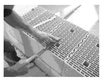
Figure 2: Ziegel walls blocks showing cellular construction [6]
